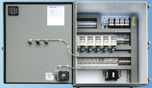
Interior: Wall Mount MCC
